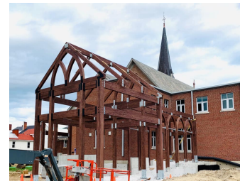
Progress continues on Cynthiana’s new West entrance renovation. September 27, 2020
